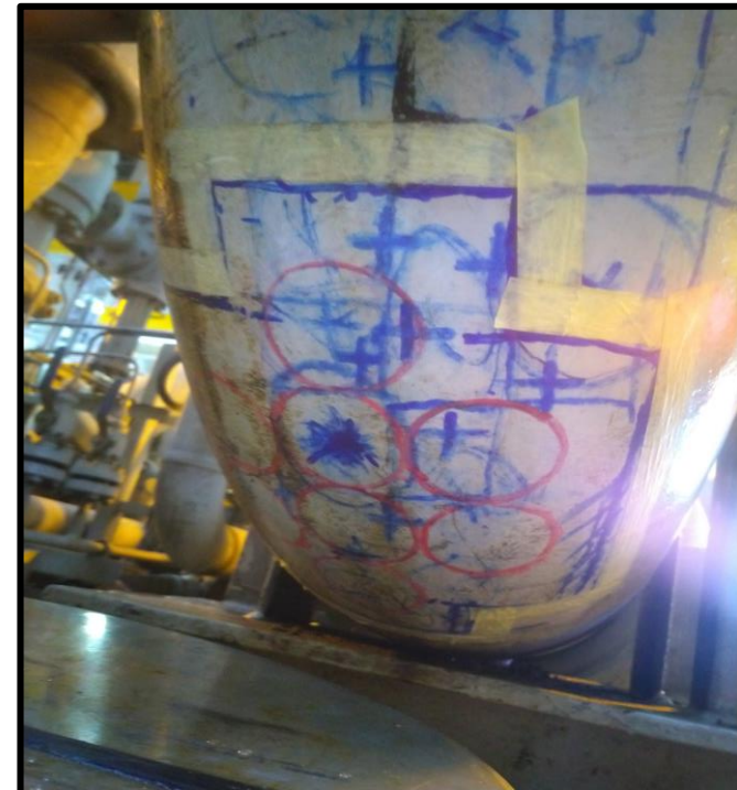
Marked out location for Sensor Installation
