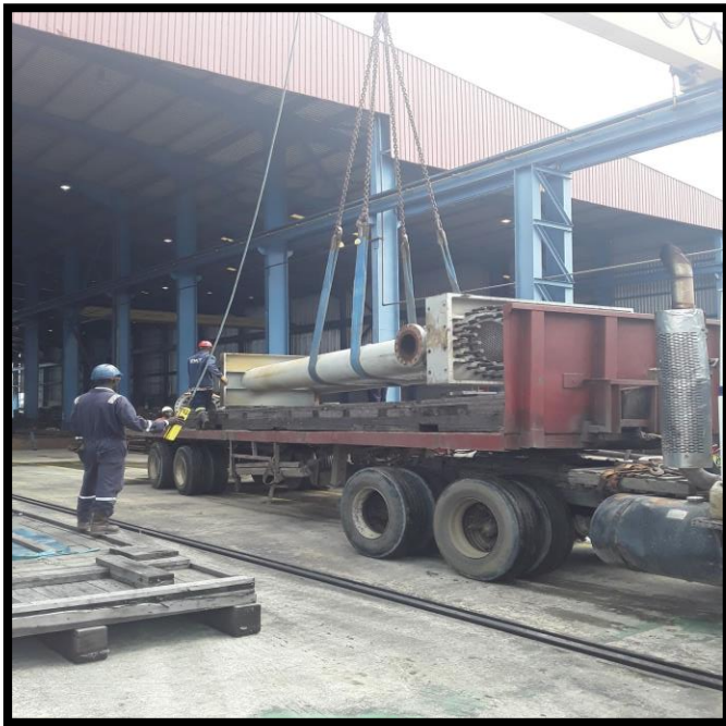
Heat Exchanger Offloading
